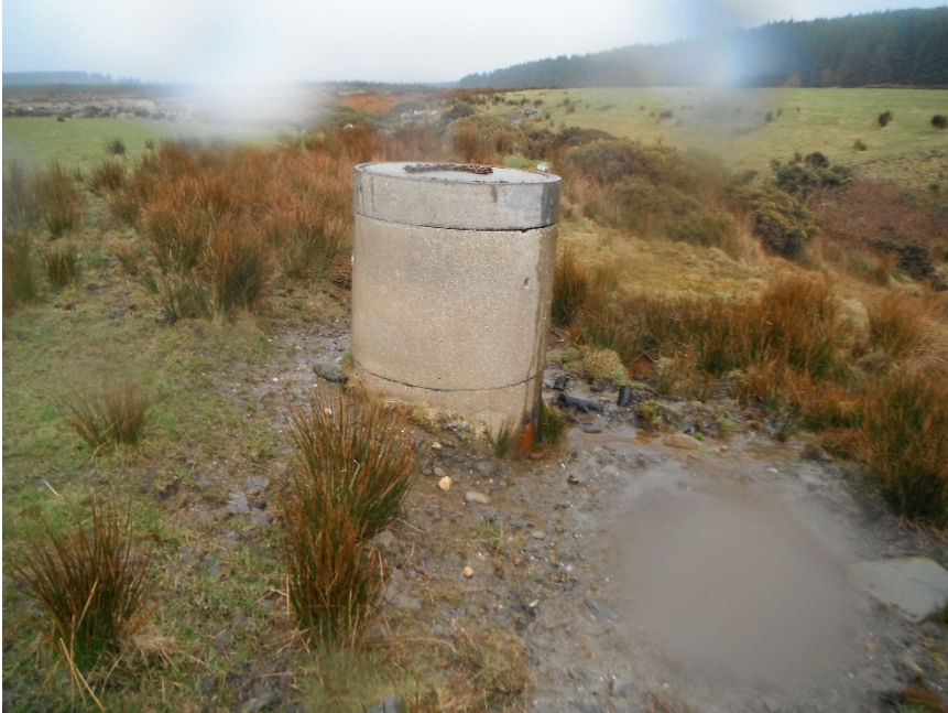
Source concrete collar and cover
