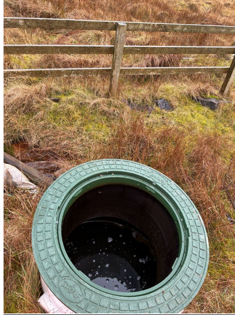
Plate 2 Tangy Farm. Groundwater spring on the existing Tangy Windfarm. Cylindrical plastic with a plastic lid and a metal covering (taken February 2026).
