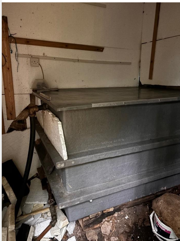
Figure 4.2: Fibreglass header tank located within uninsulated shed.
