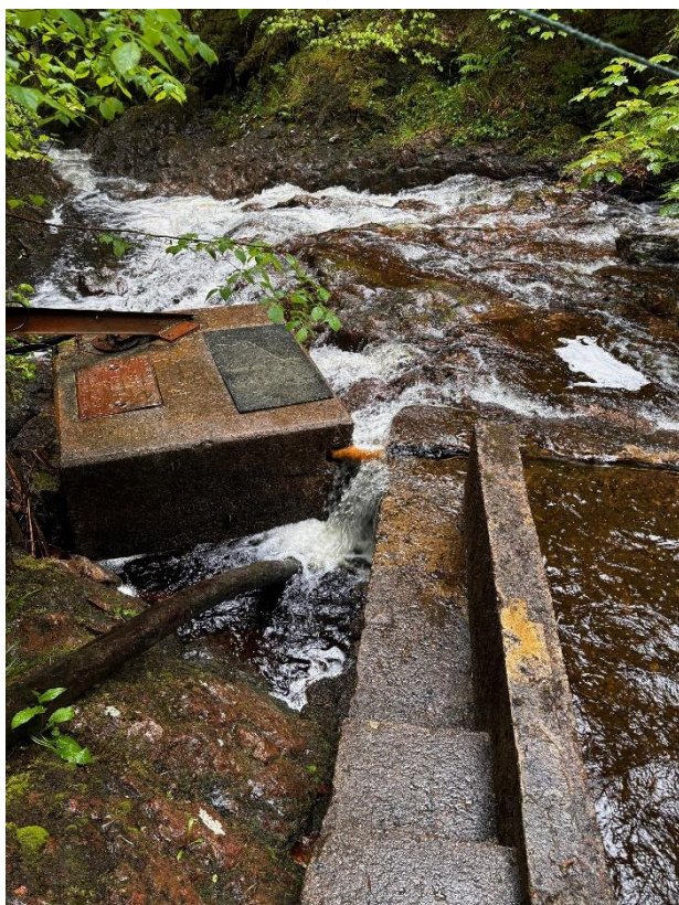
Figure 4.1: Surface water inlet in the Allt Sigh watercourse showing dam feeding the capture tank via an open pipe.
