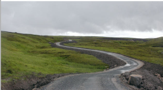
Floating track construction - Glendoe Hydroelectric scheme
